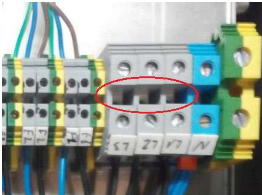
Figure 3.2: Three-phase connection
