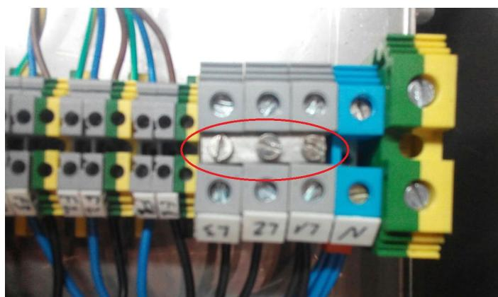
Figure 3.1: Single-phase connection
