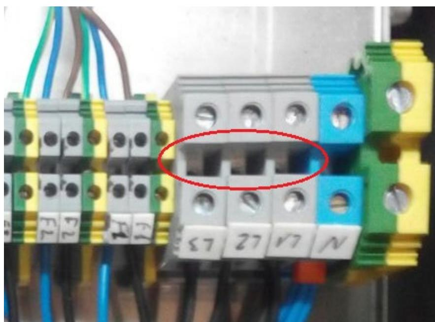
Figure 3.2: Three-phase connection
